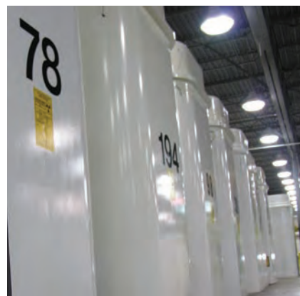
Figure 7.26 Each of these 450 containers holds nuclear waste from the Pickering, Ontario, nuclear power plant. About 40 new containers are added each year. Each container is designed to last for about 50 years while a long-term storage solution is sought.
